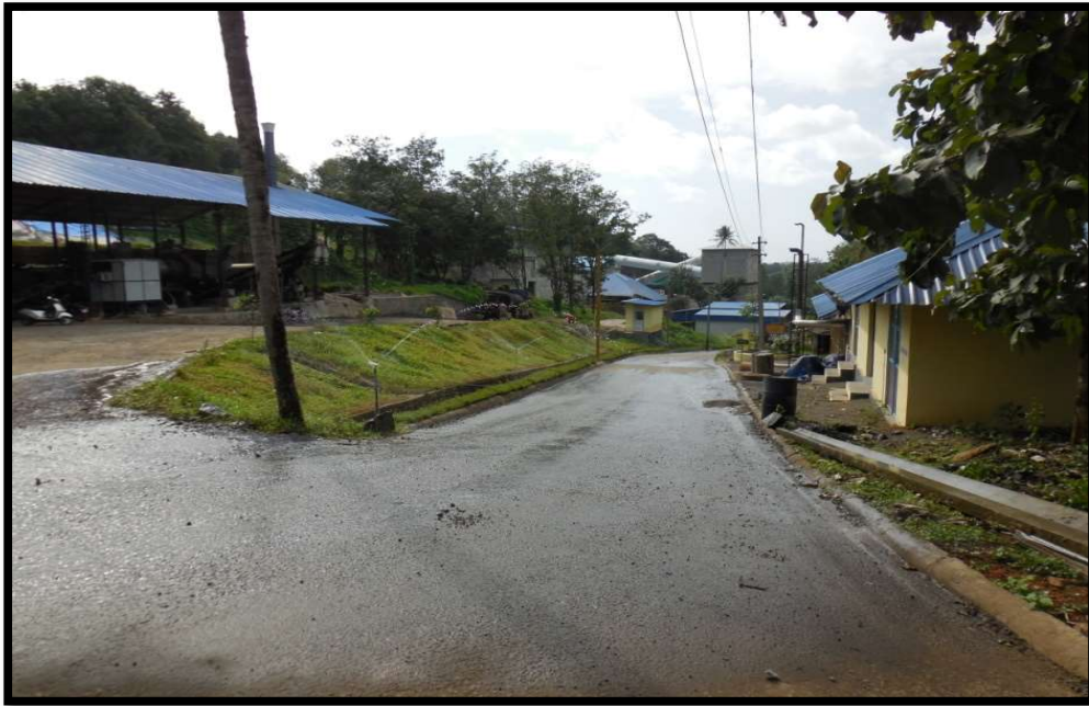
Sprinklers installed in the project site
