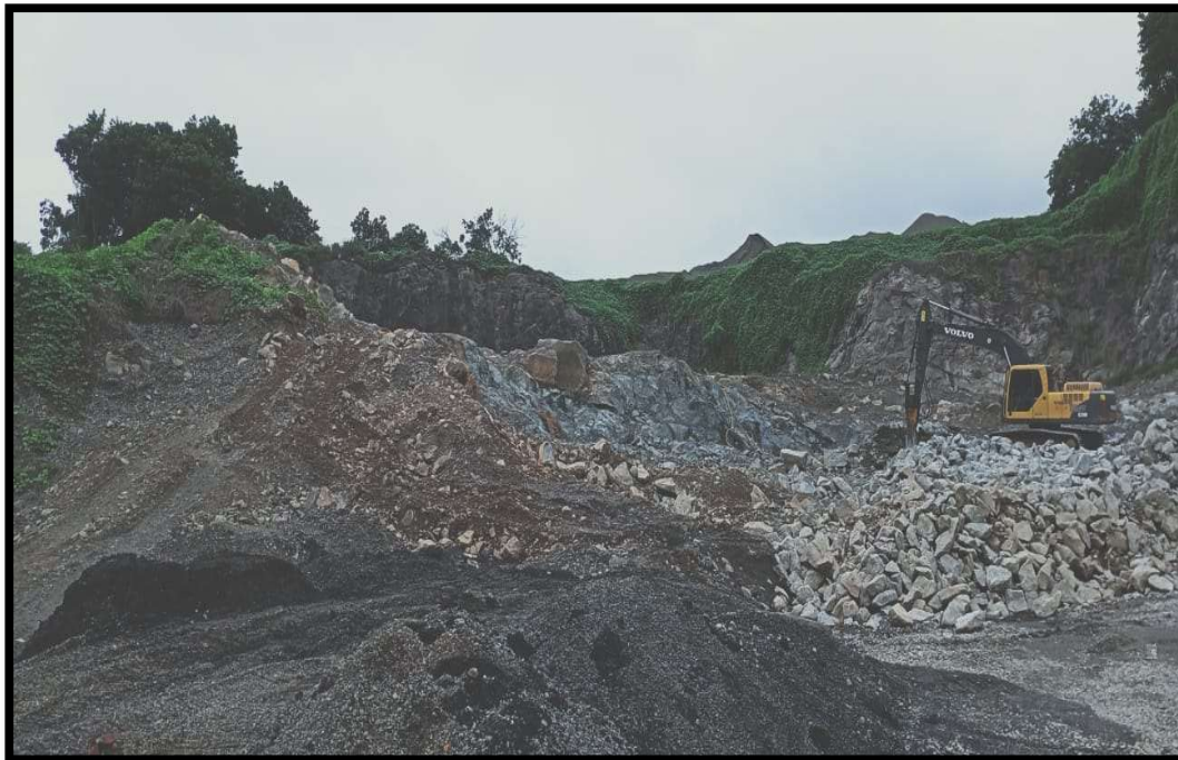
Bench system is progressing
