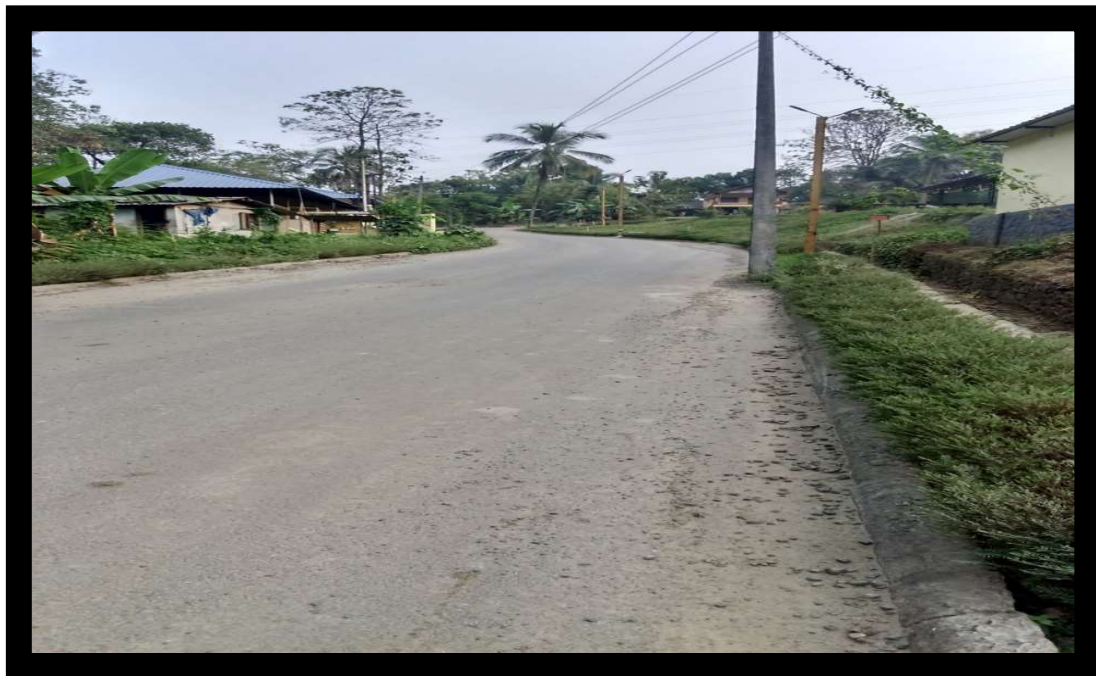
Tarred road to the Quarry
